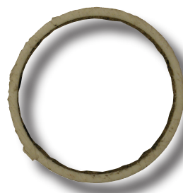
Cooling water pipes after less than one year's operation with Tekleen filtration.
